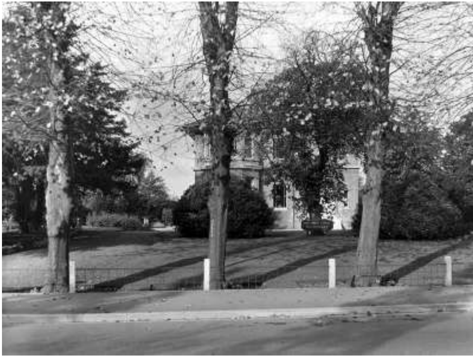
Front of High Trees as shown on the Baker Perkins site (c1950s)
